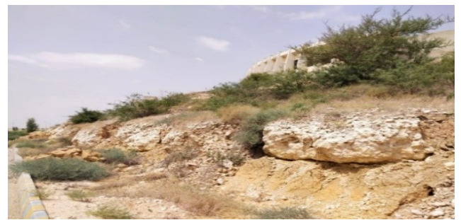
Fig. 1.2 Site Slope A of investigation.
